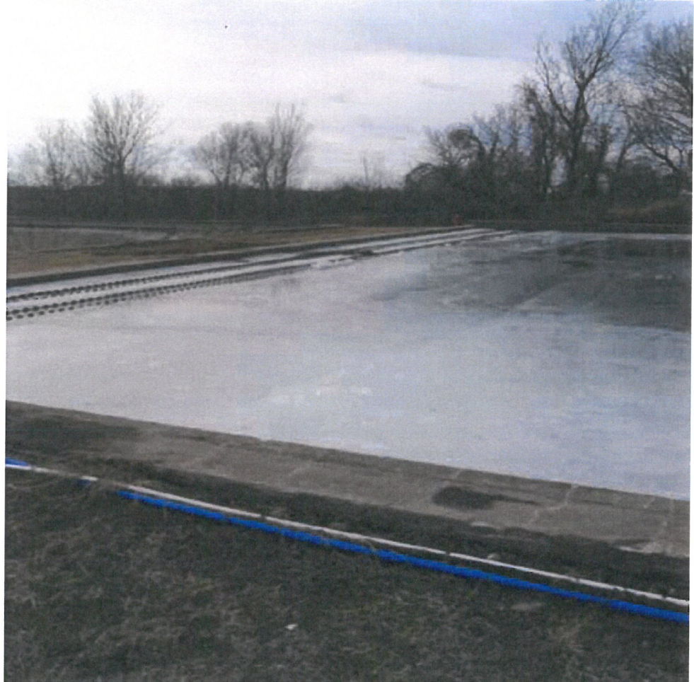
Pre-sed Clarifier Basin
