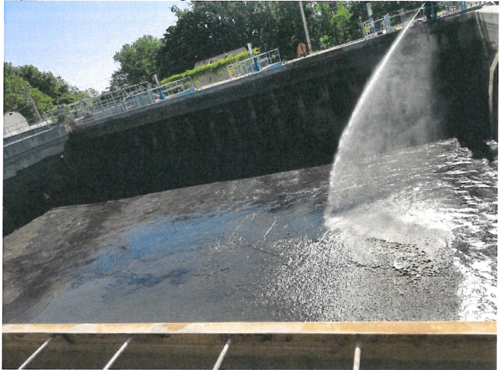
Square Section Cleaning
