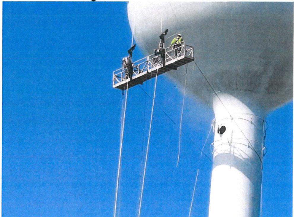
Water Tower Painting
