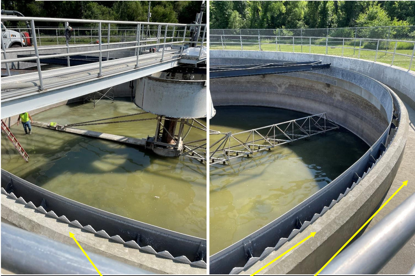
Clarifier #1 walls and trough concrete repair performed by Smi-co
